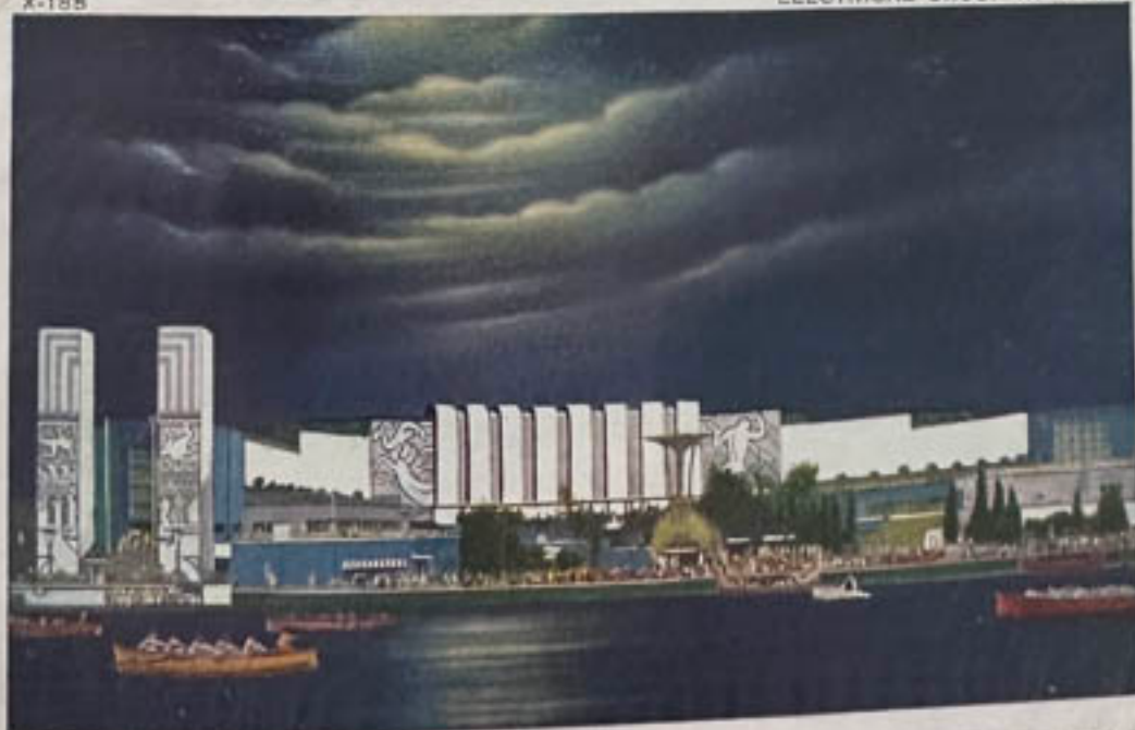
ELECTRICAL GROUP AT NIGHT
