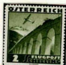
RAILROAD VIADUCT, CARINTHIA
