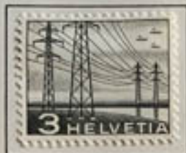
328 High Tension Wires
