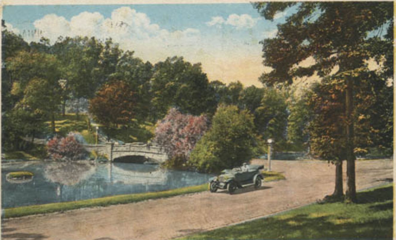
STONE BRIDGE, LINCOLN PARK, SPRINGFIELD, ILL.
