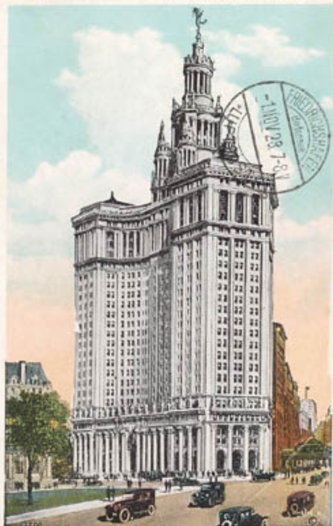
512.—THE MUNICIPAL BUILDING, NEW YORK CITY.
