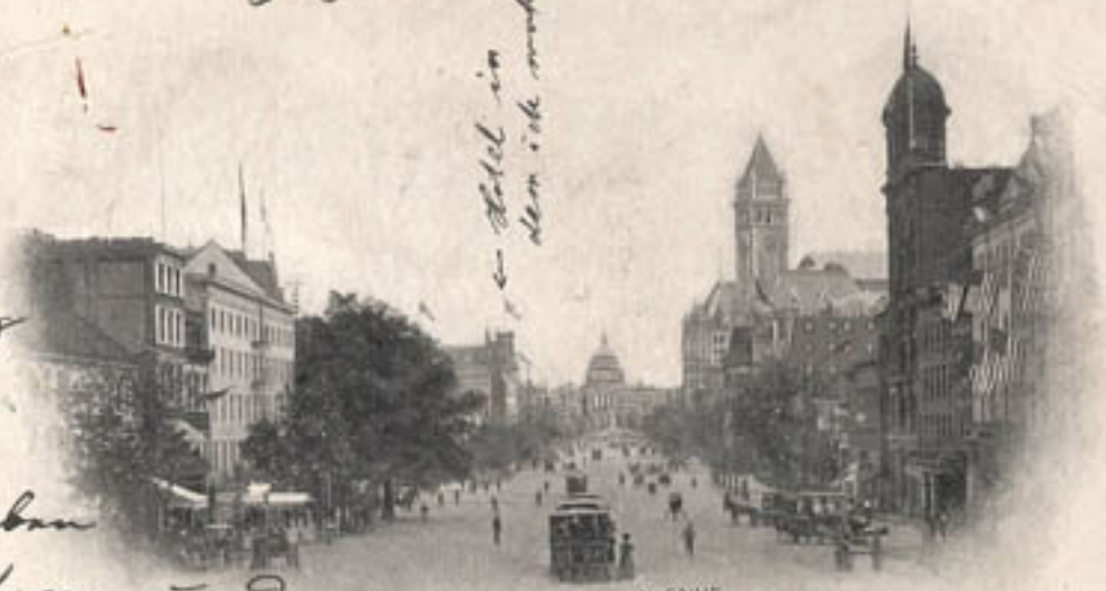
PENNSYLVANIA AVENUE FROM TREASURY BUILDING WASHINGTON, D.C.
