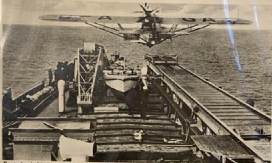
10 ton Dornier Mail Flying Boat catapulted from the Lufthansa Floating Base MS „Schwabenland“ in the South Atlantic
