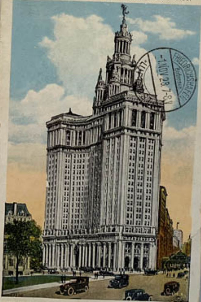
112.—THE MUNICIPAL BUILDING, NEW YORK CITY.
